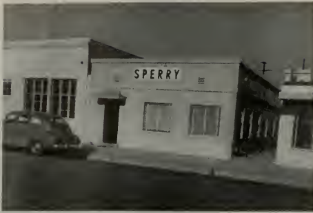
Sperry's marine branch office at 128 No. Marine Avenue, Wilmington.
